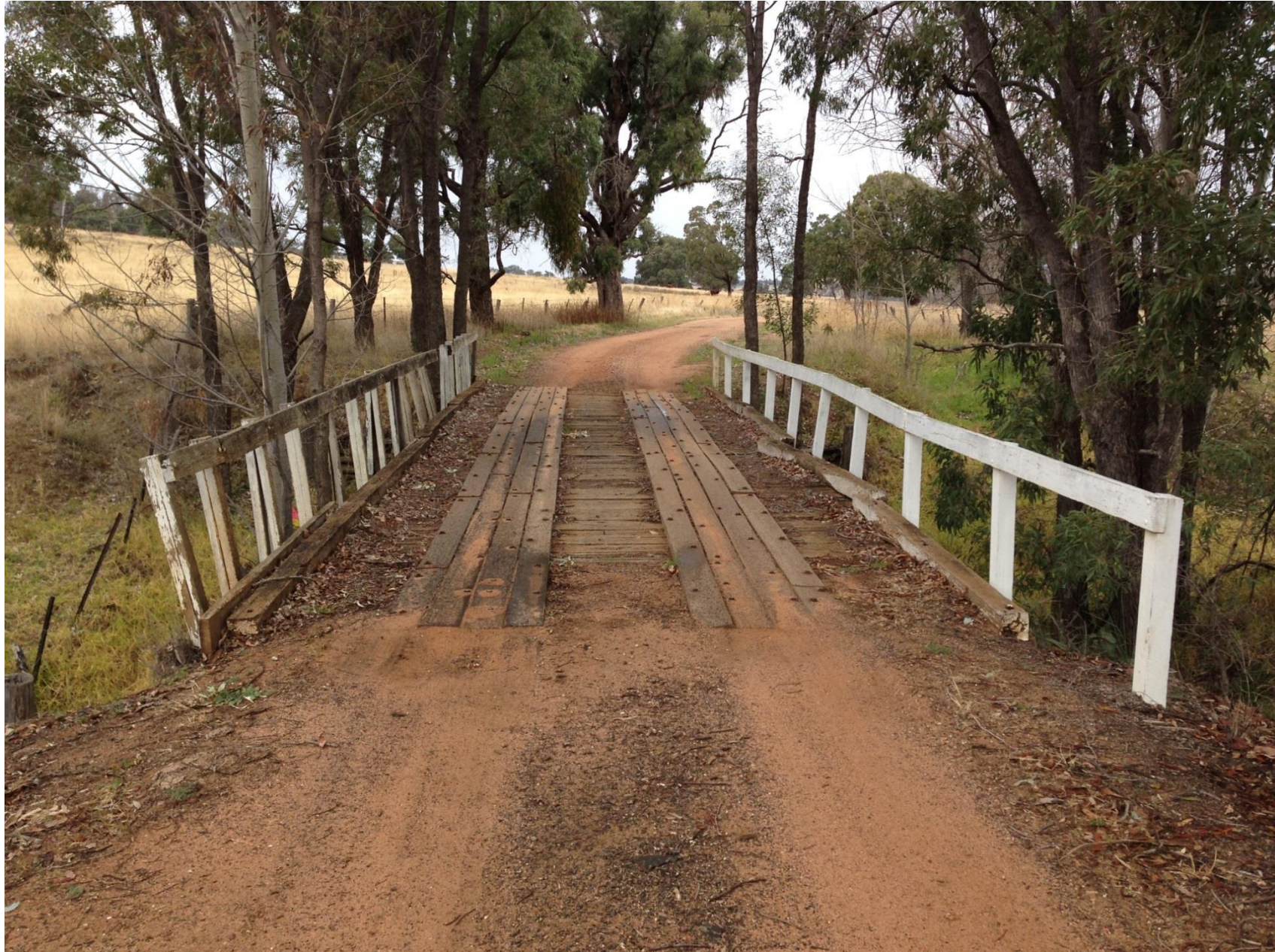
Coonagoony Bridge on Elah Road.
