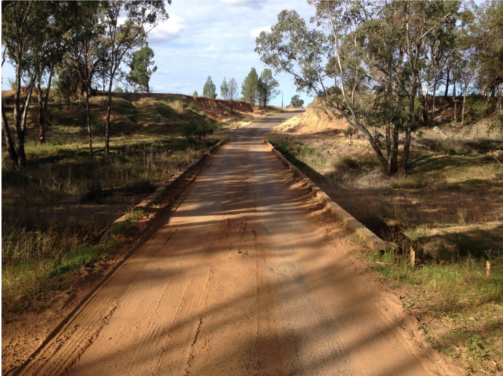
Bridge over Baradine Creek near the Village of Kenebri.
