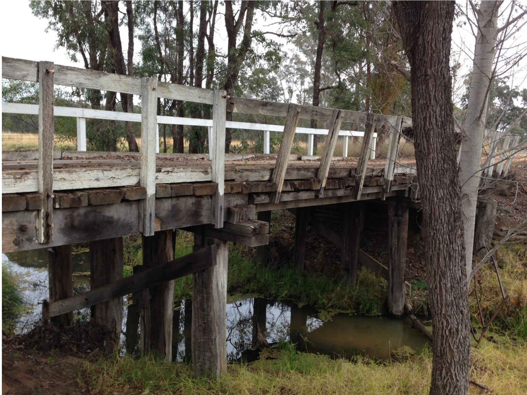
Side view of Coonagoony Bridge.
