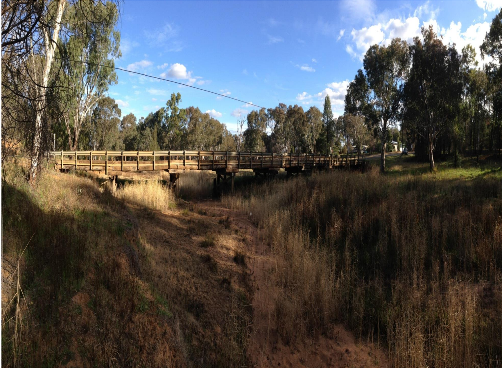
Baradine Creek Bridge – View of timber bridge looking upstream.
