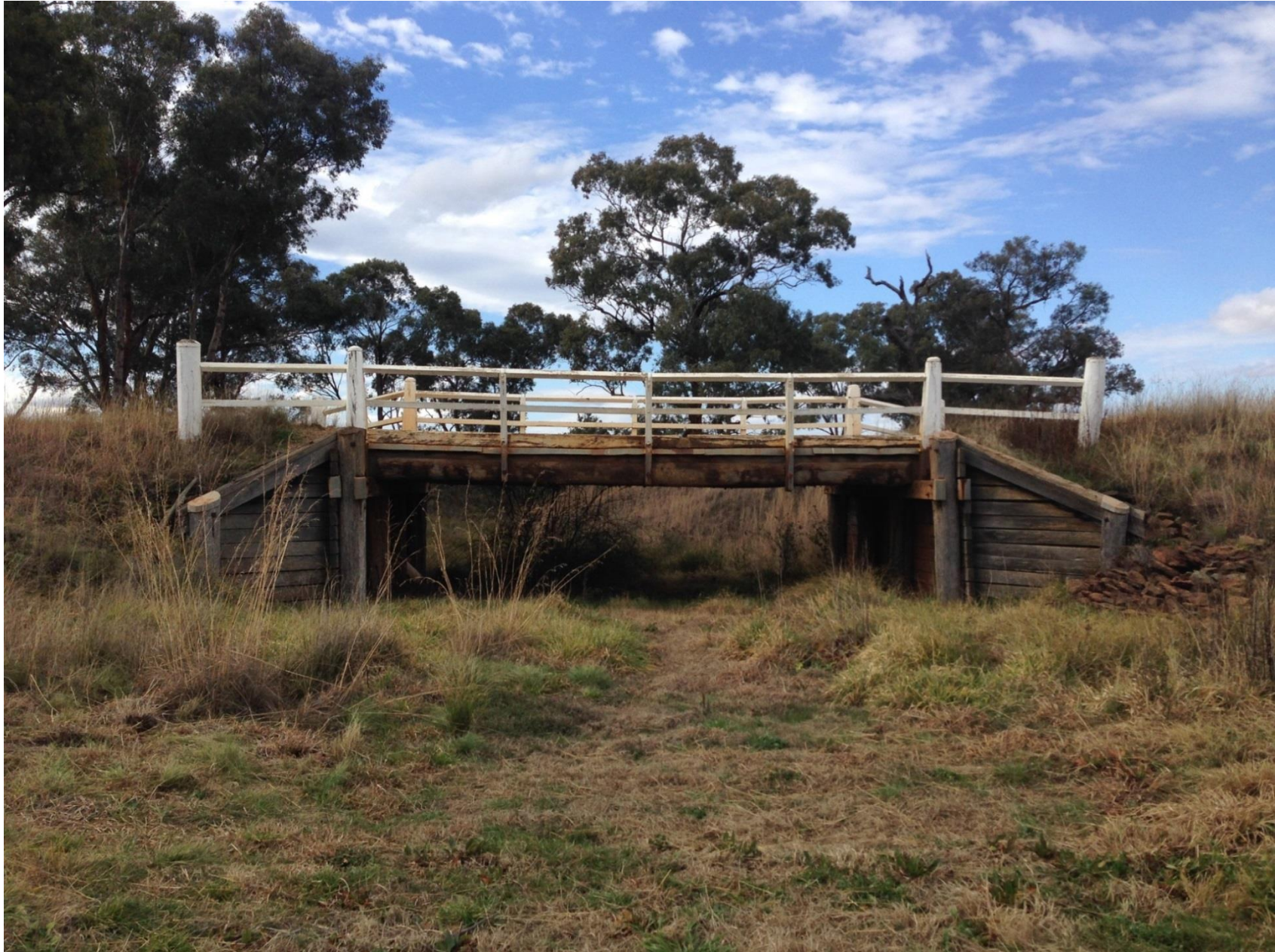
Side view of Black Gully Bridge on Leaders Road.
