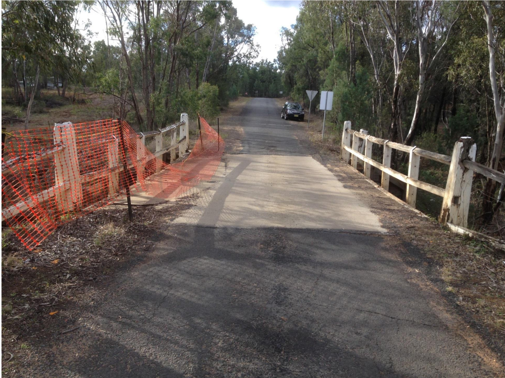
Existing timber bridge over Worrigal Creek on Aerodrome Road, Baradine.
