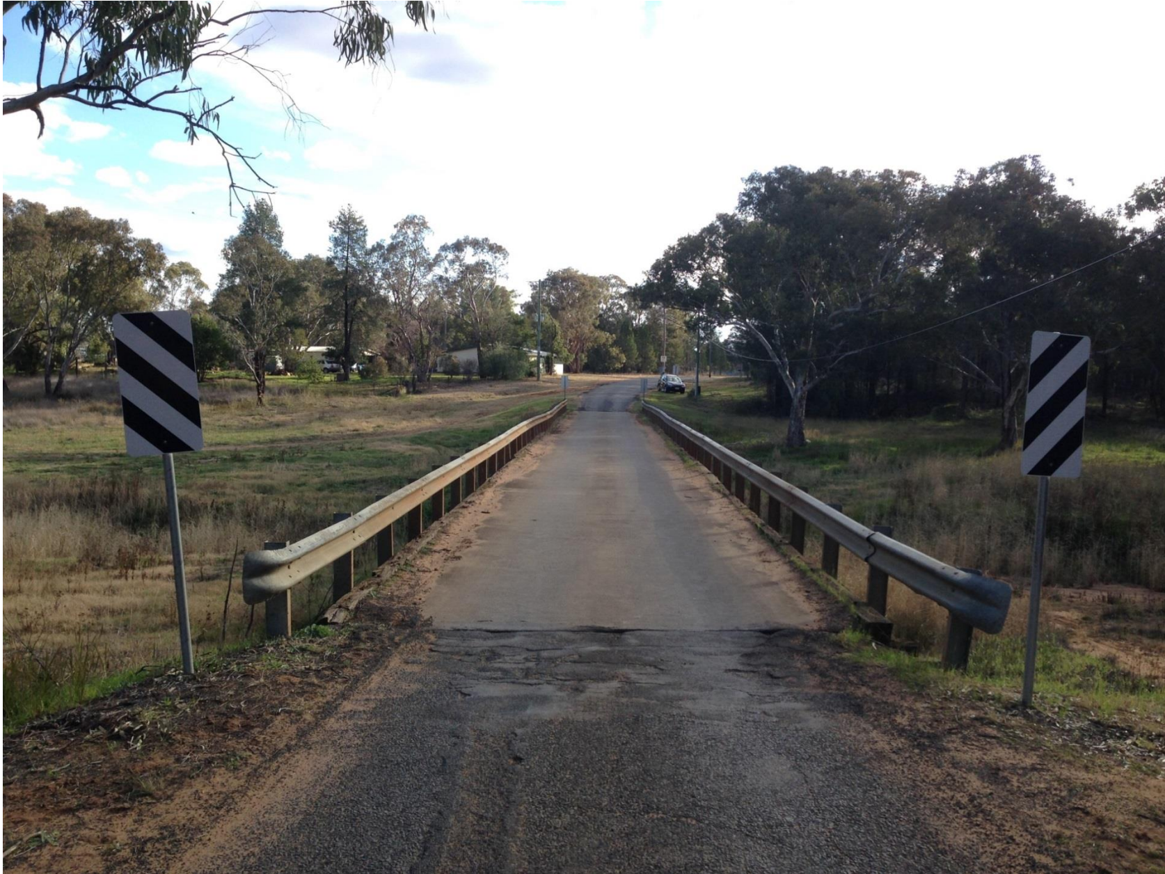
Baradine Creek Bridge in the town of Baradine.
