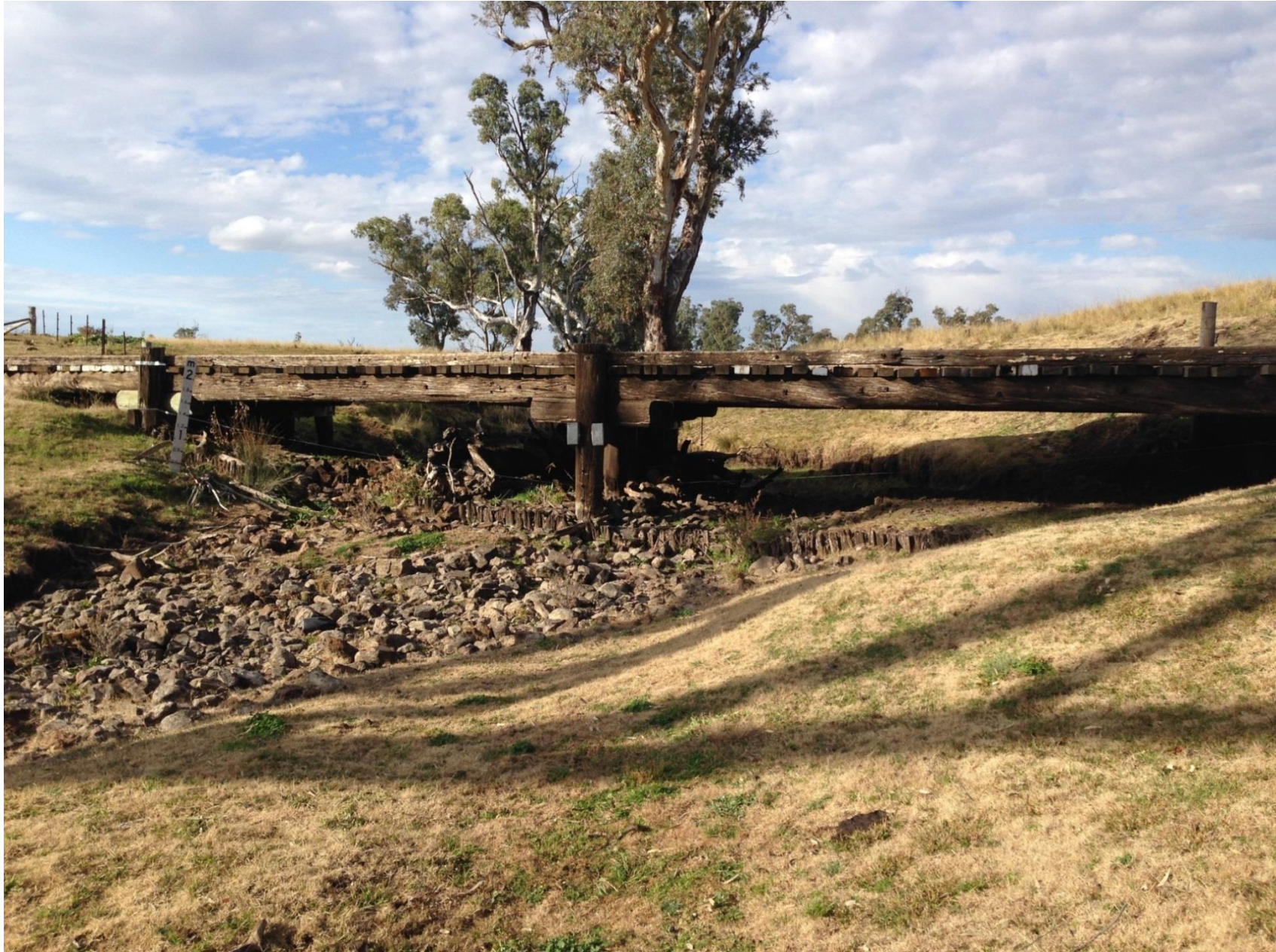
Side view of Ross Crossing timber bridge over the Talbragar River.
