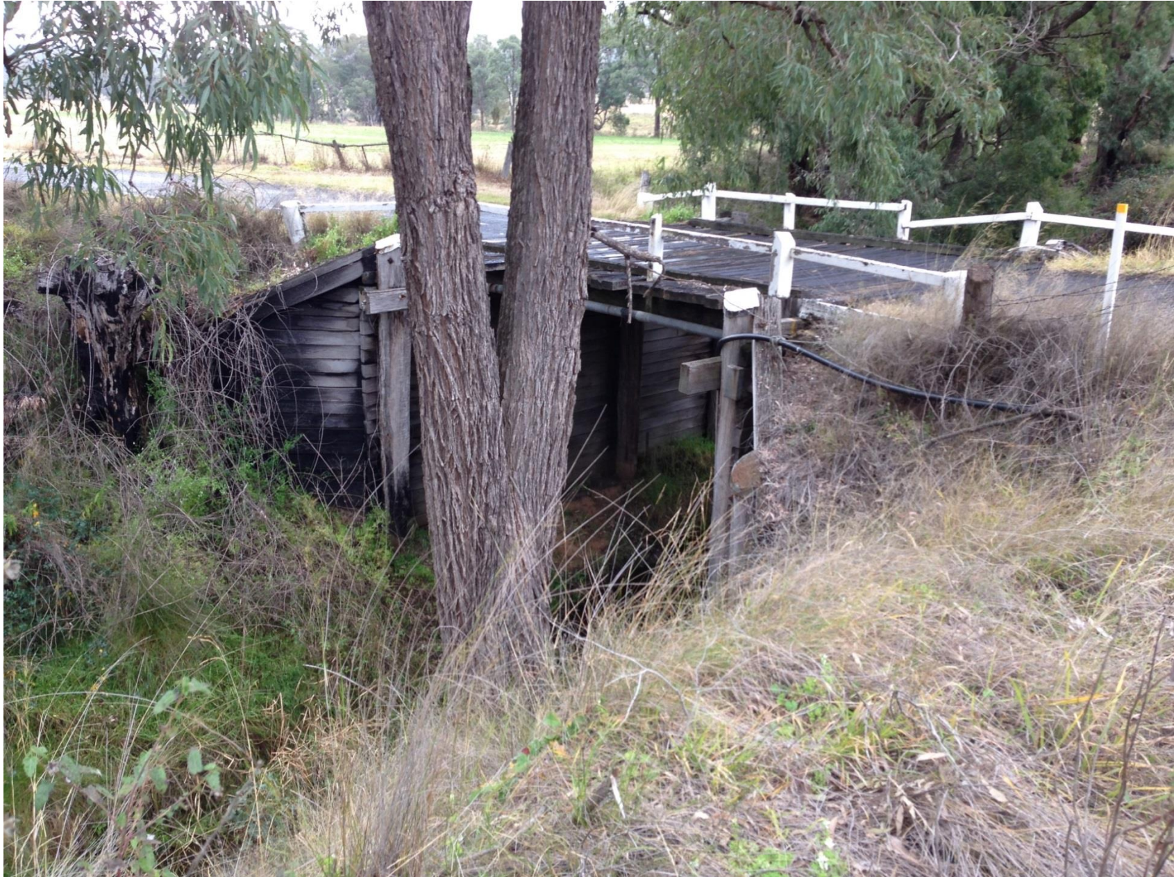
Side view of Warkton Bridge.
