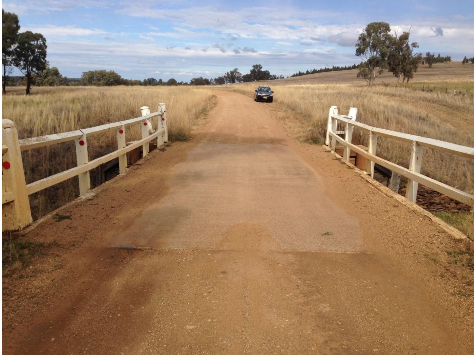
Black Gully Bridge on Leaders Road provides freight access to farming properties adjoining the Castlereagh River near Binnaway.
