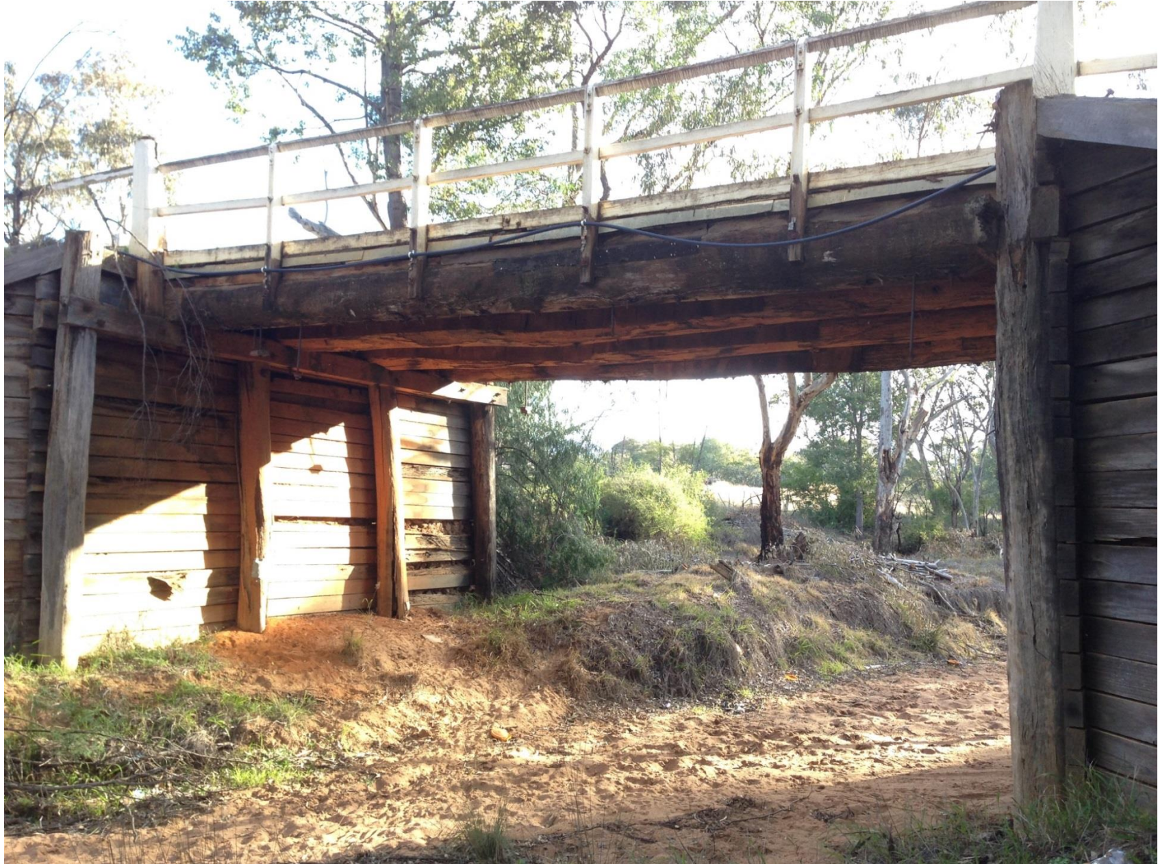
Existing timber bridge over Worrigal Creek.
