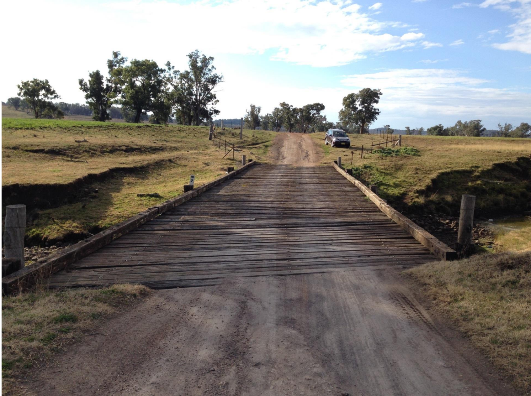
Ross Crossing timber bridge over Talbragar River on Blue Springs Road.
